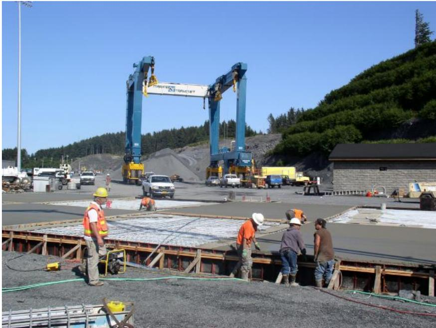
By comparison, an empty Marine Travelift 600C weighs 275,000 pounds more than an empty 747-400 jumbo jet. When lifting its maximum capacity, the lift's total weight reaches 2 million pounds, compared to 910,000 pounds for the heaviest fully loaded 747. "We had to build a one-foot reinforced concrete wash-down pad to the specs for landing a 747," explained Owen. "And, we are fully compliant with all environmental requirements."
